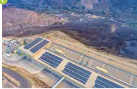
Dry fermentation for household waste and organic waste Santa Barbara (US) 67,000 t/a Year of construction 2020
